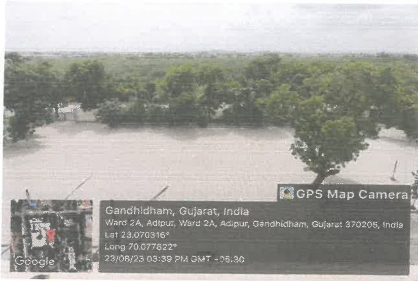
Renovation – Ground- Paver Block
